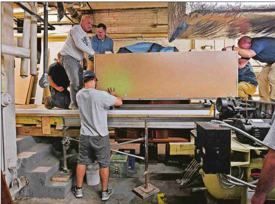
The team moves the sculpture carefully under low ductwork and across a bridge in the museum's boiler room, on Monday.
